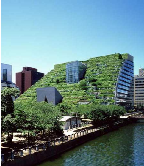
Figure 4.1 Green roof in Tokyo ( www.greenroofs.worldpress.com ).
